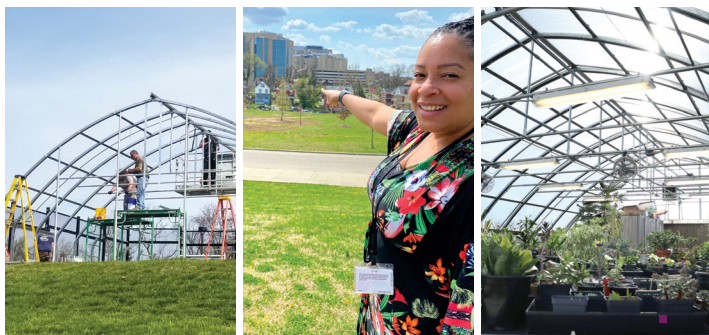
L to R: Crews dismantle the greenhouse at Cincinnati Children's College Hill location. Dr. Jaren Finney, Rockdale Principal, points to where the greenhouse and Urban Learning Garden will reside. Inside the greenhouse during years at the College Hill location.
